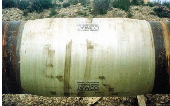
Figure 3: Composite crack arrester used in the Demopipe project
