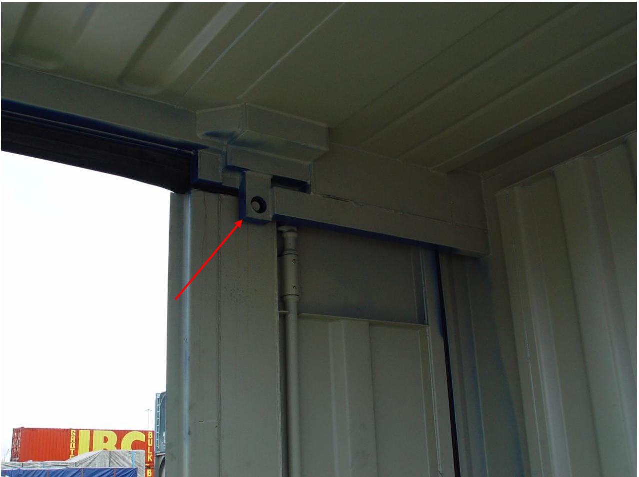
Figure 5. Top of one of the side doors (view from inside container) showing the top pin still connected to the 40ft. casting.
