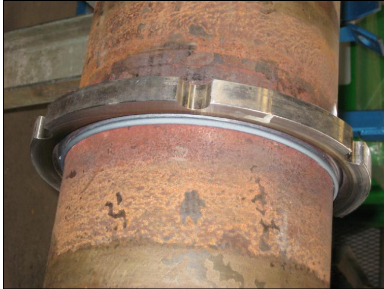
Figure 5. Visual examination of weld 2
